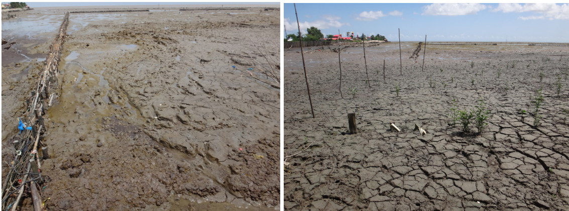
Figure 20.37 Evolution of the mud deposit of the sediment trapping unit at Weg naar Zee: situation in April 2016 (left) and June 2017 (right). (Credit: S. Naipal)
