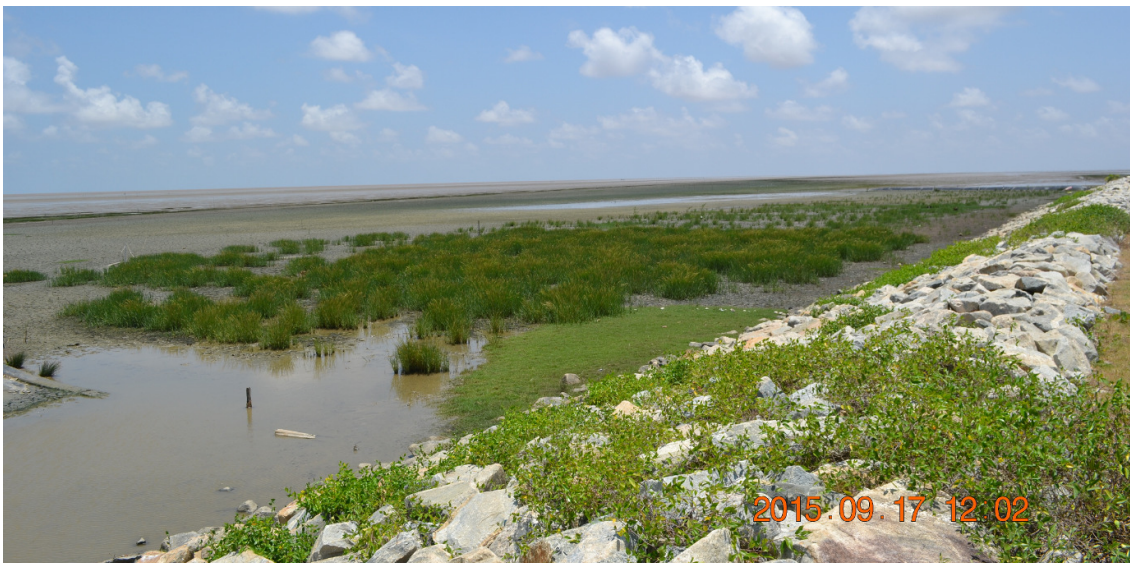
Figure 20.33 Top: Devonshire Castle shoreline (Guyana) was planted with Spartina in May 2015 following construction of geotextile tube. Bottom: Rapid colonization of Spartina within five months. (Credit: R. Adams, NAREI)
