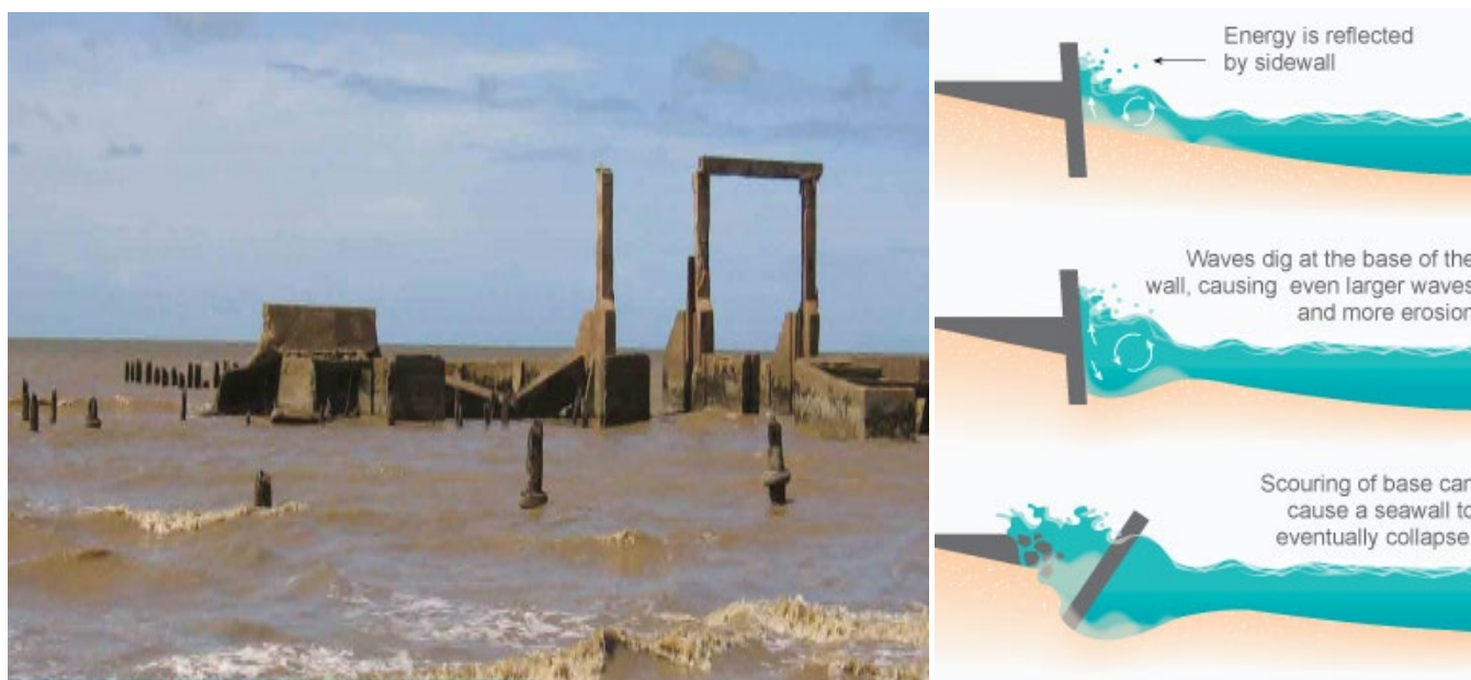
Figure 8. Failure of hardened sea defense structure in Guyana
