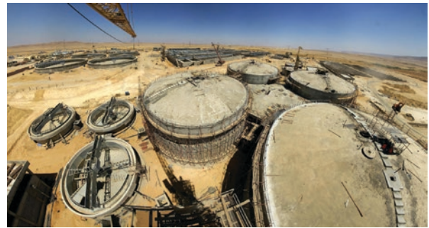
PHOTO 1. New Cairo Wastewater Treatment Plant
