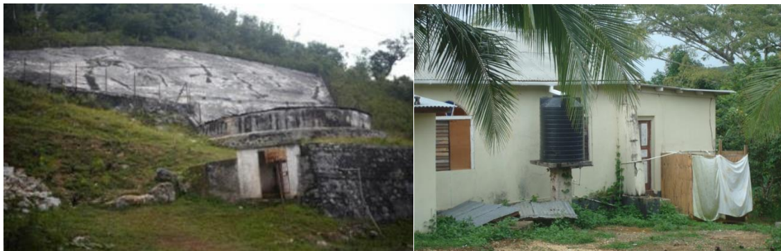
Figure 7.2: Community and Household Rainwater Harvesting System in Jamaica
