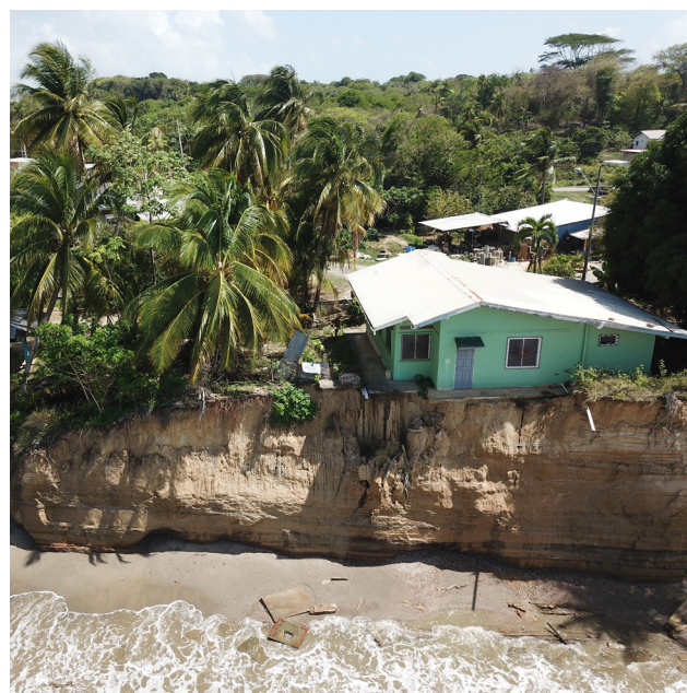
Coastal erosion in Guayaguayare, South Trinidad, May 2018.
